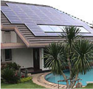
Side view of the bio-solar house designed and occupied by Soontorn Boonyatikarm, professor of architecture at Chulalongkorn University in Bangkok. Photo: Soontorn Boonyatikarm
